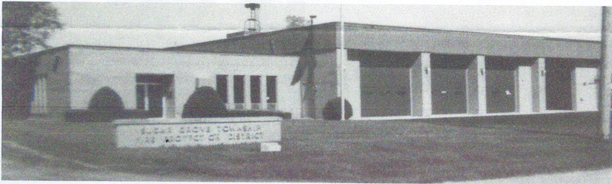
The fire department moved to the north end of Main Street in August 1973. It was still a volunteer Fire Department with 35 members. It was run for many years without raising the tax rate.
